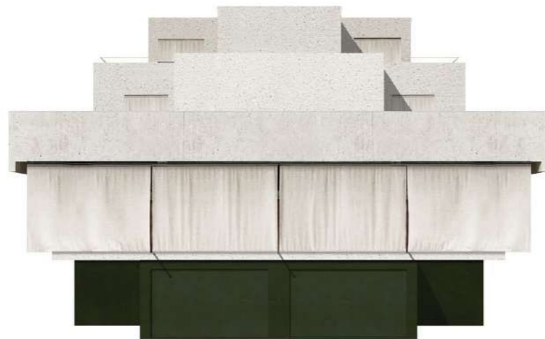
Residential building – Oberwil
